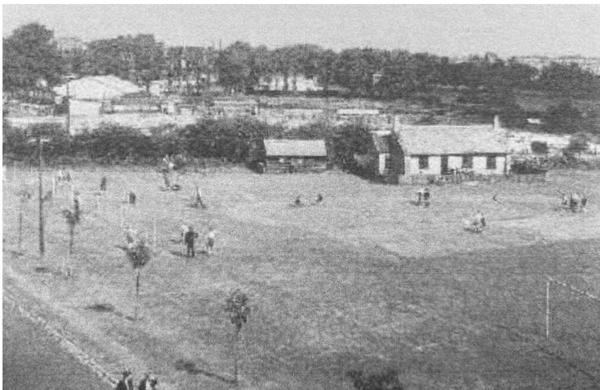
Beyond Gilbert Cottage in Gilbert Lane is Home Park being re-built. The original wooden grandstand is demolished and the roof over the Devonport end is up. Cutting across the bottom left corner is the old pathfield from Pennycomequick just prior to being widened and surfaced in the conversion of farmland into Central Park. Along it new trees have recently been planted. To the right is a goal post of Higher Home Park (Cottage Field) circa June 1930.
