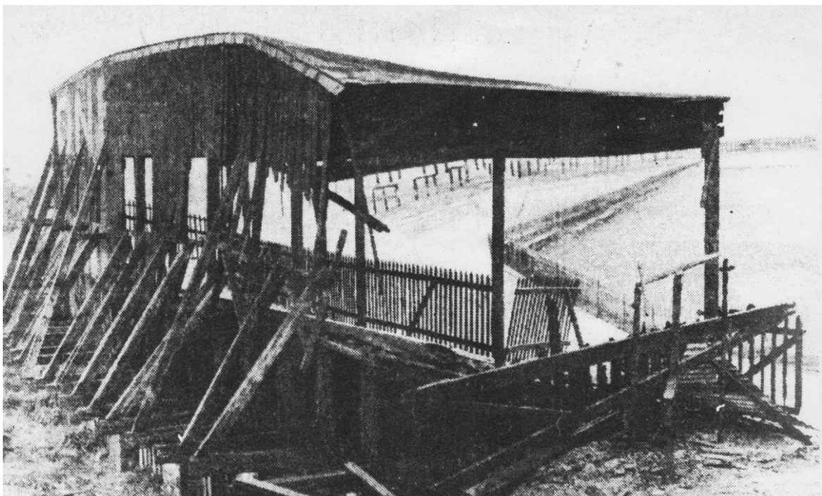
The thirty-year-old wooden Flower-pot stand was the victim of the first fire at Home Park. After a match (no pun intended) a fire was spotted, thought to have been caused by a smouldering cigarette. It was doused before the stand was totally destroyed. The burnt timbers were cut away and after repair it continued truncated. In fact, what remained was to survive longer than the new grandstand opposite to it. (Western Morning News, 24 th April 1933).
